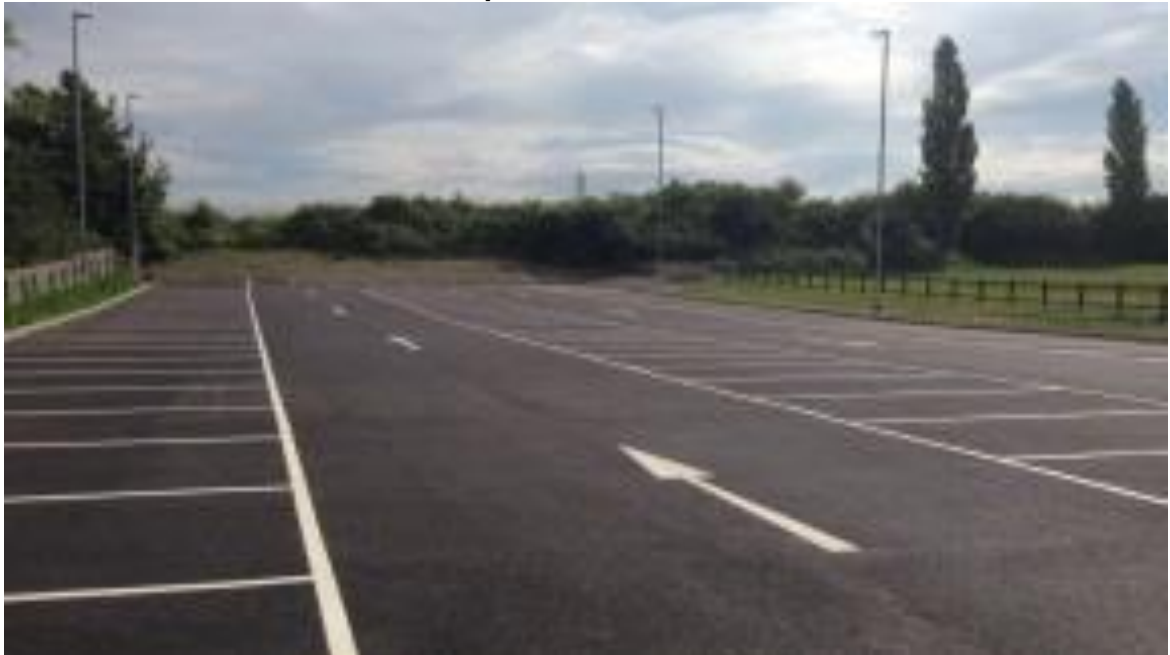
Completed Car Park
